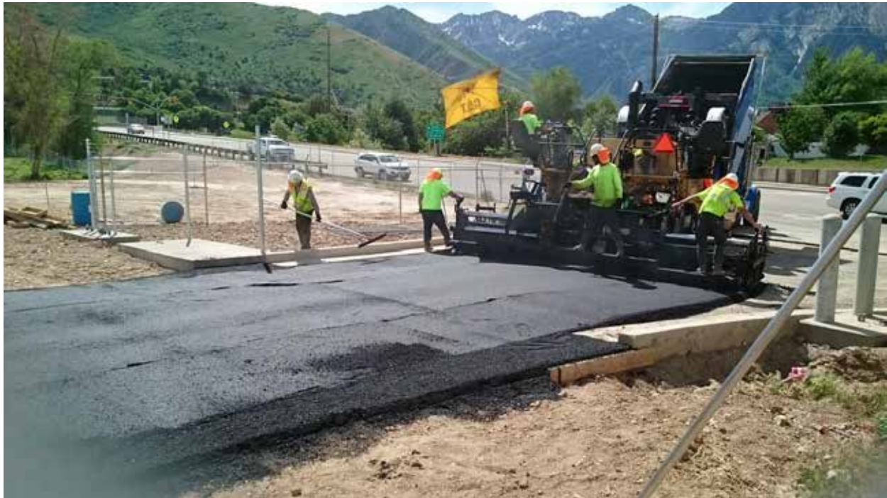
Asphalt work was completed around the site.
